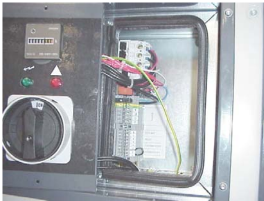
The terminal strip is located behind the control panel at the right hand side of the unit
